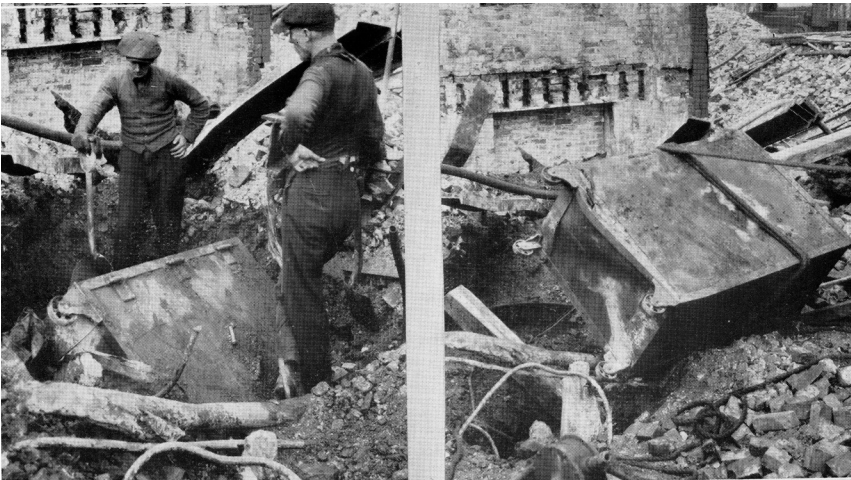
During a fire, a UL-labeled safe dropped from the sixth floor to the basement of a building. The safe contents were then checked for damage and found to be in normal condition (1922).
