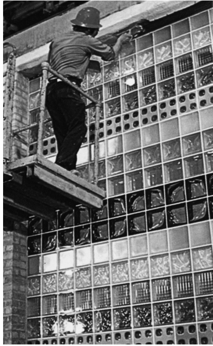
A UL technician prepares a glass block wall for a fire test (1977).
