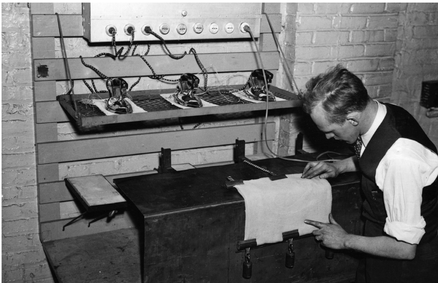
Electric irons and heating pads are tested for their flammability risk (1937). Photograph credit: Associated Press
