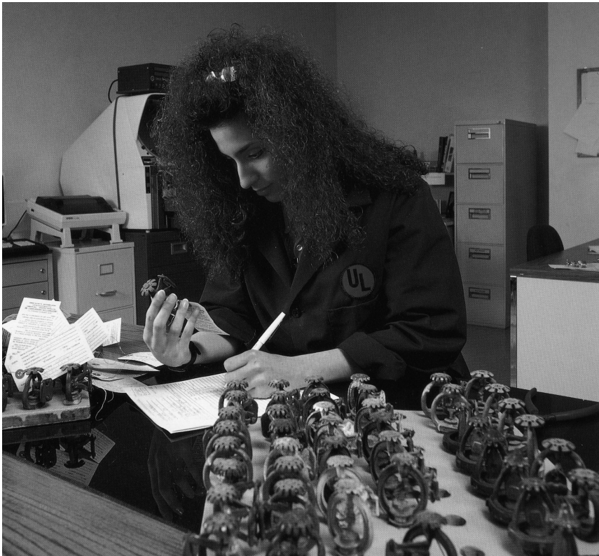
A technician examines each sprinkler sample before it is subjected to any tests (1992).
