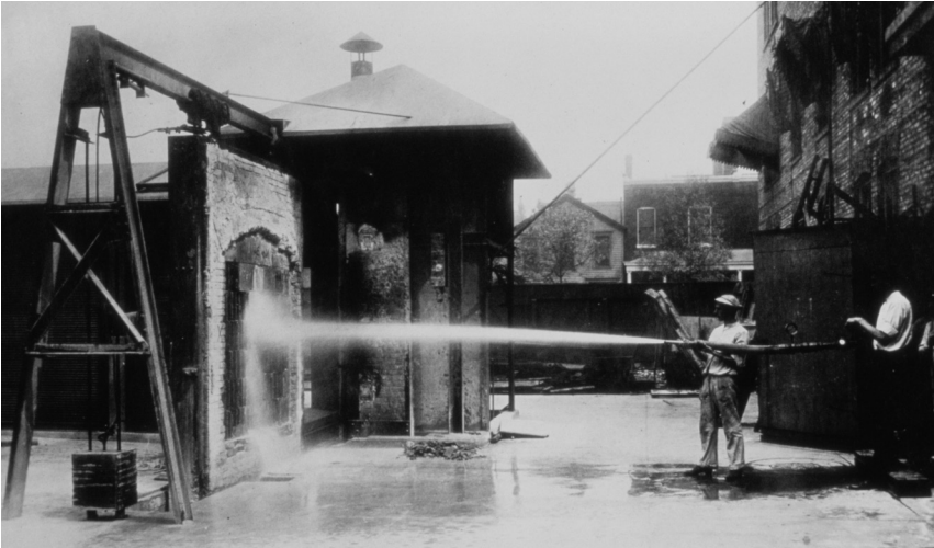
After removing a fire door from a testing oven, UL employees subject the door to a hose stream test (1915).
