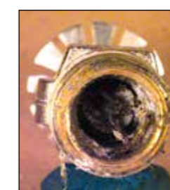
Figure 2: Photograph illustrating the level of deposits commonly found in sprinkler inlets.
