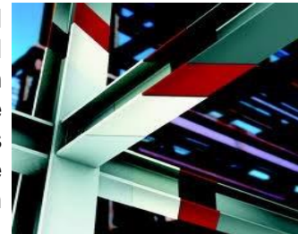
Figure 3 – Steelwork Fire Protected By SFRM Coating System (Photo Courtesy Of GCP Applied Technologies)
