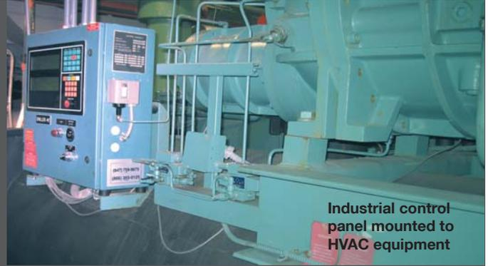
Industrial control panel mounted to HVAC equipment
